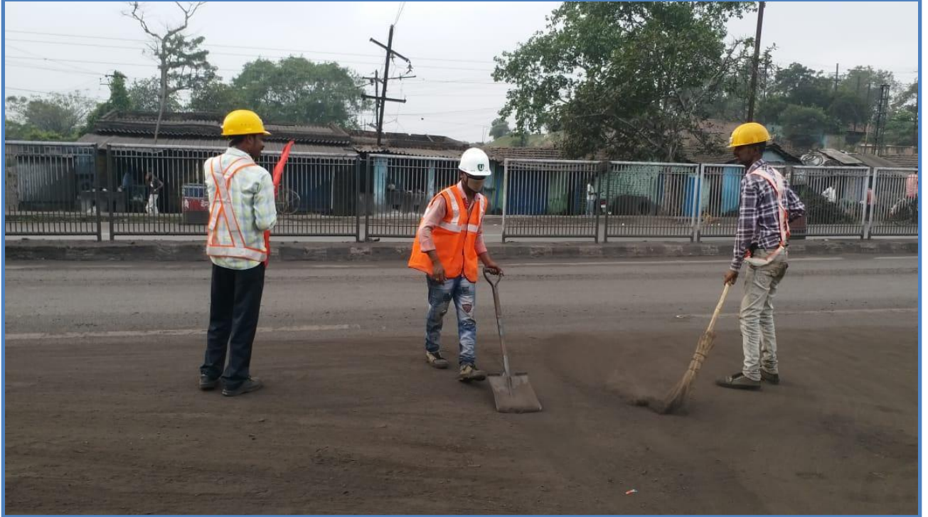
Picture 2 – Road Cleaning (Mechanical Sweeper and Manual Sweeping)
